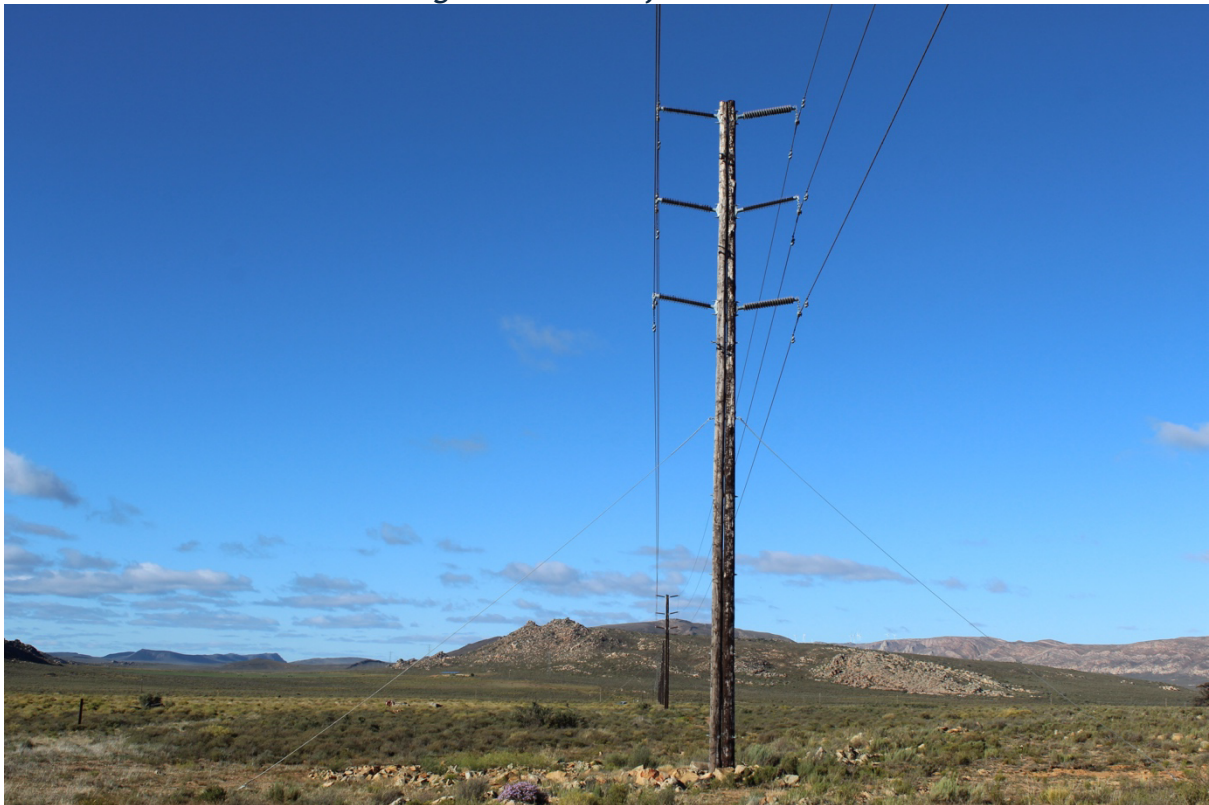
Figure 6: Wooden Towers to be replaced by Monopole Towers
