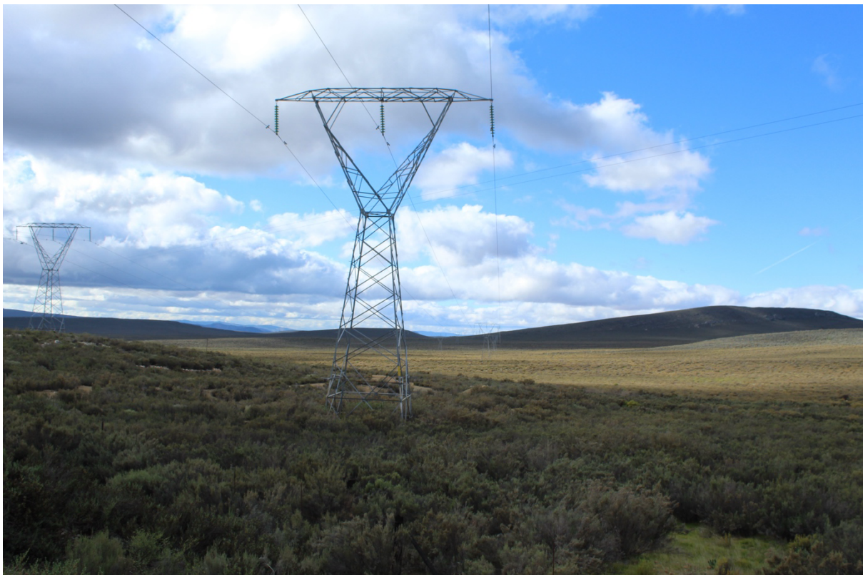
Figure 4: Picture showing the vegetation along distribution line
