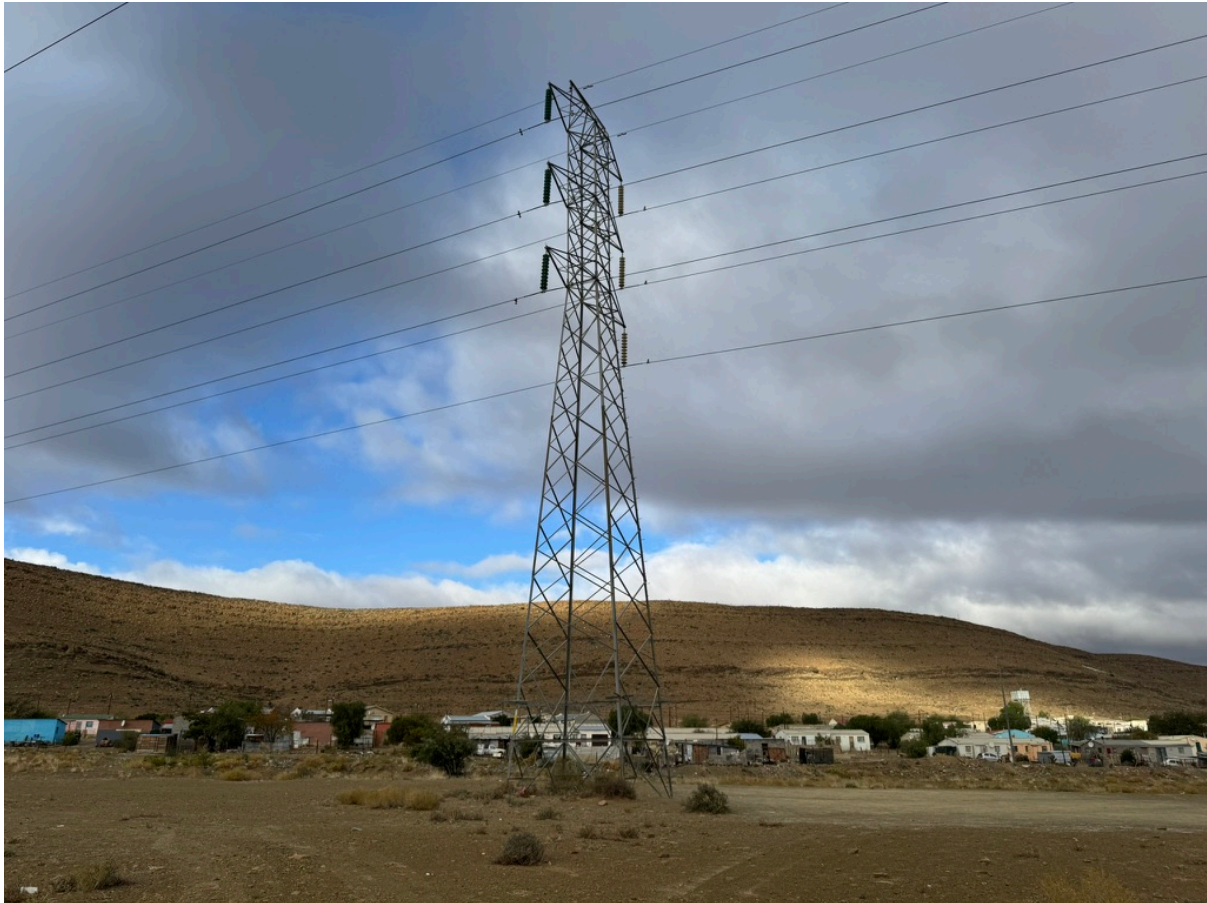
Figure 3: Lattice Tower Structure
