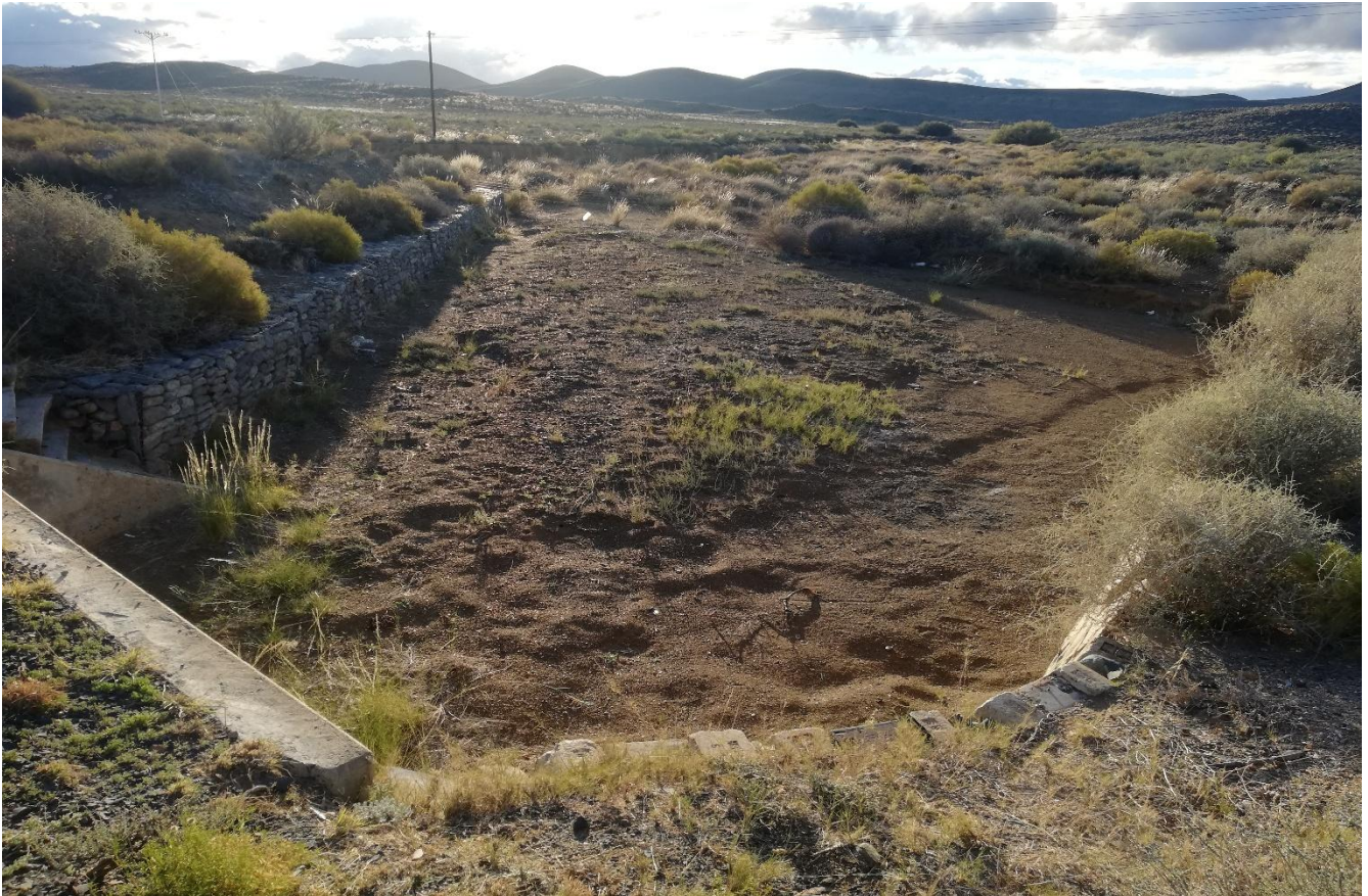
Figure 38: Baviaans River tributary culvert along the N1
