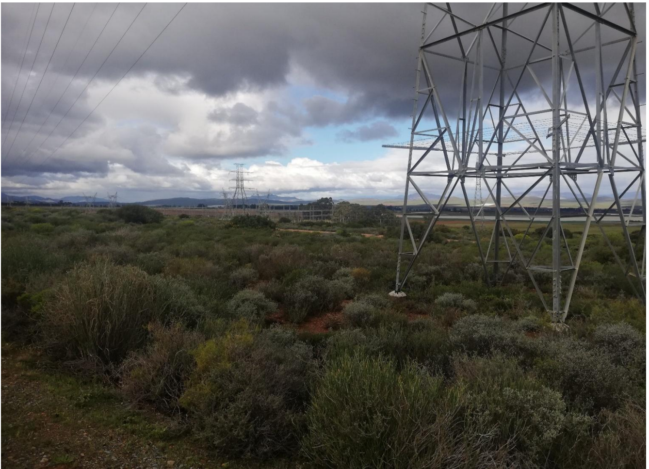
Figure 27: Photograph of the Boskloof Sub-station
